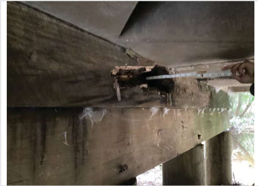
Bent 1 cap A rear side
