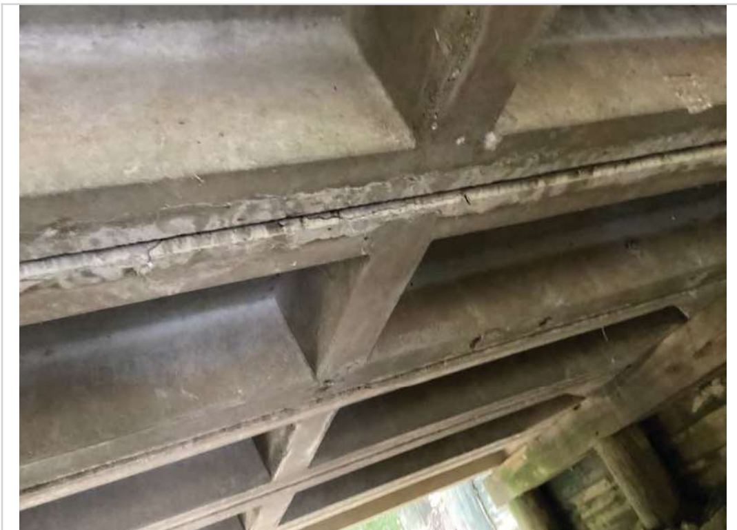
Span 2 bottom deck
