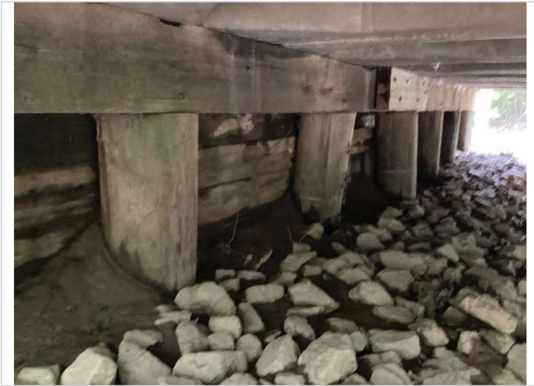
Abutment 2 cap looking ahead
