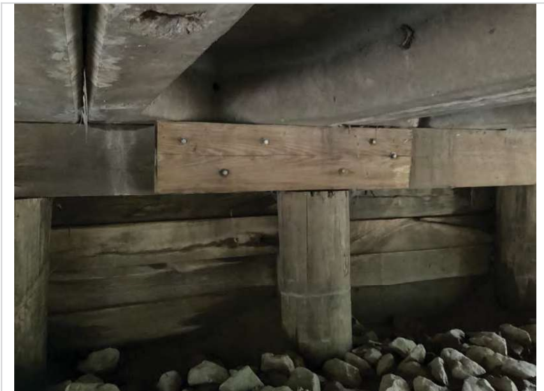
Abutment 2 above pile D
