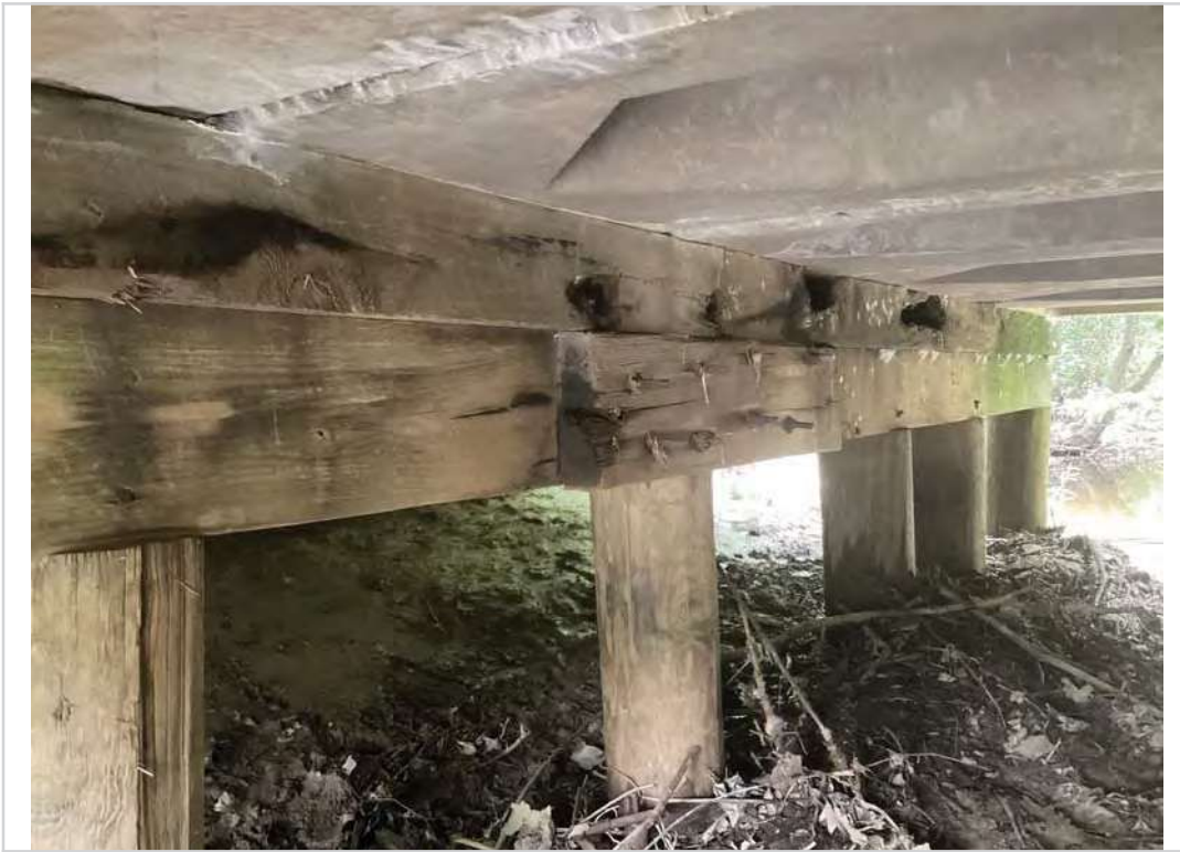
Bent 1 rear side
